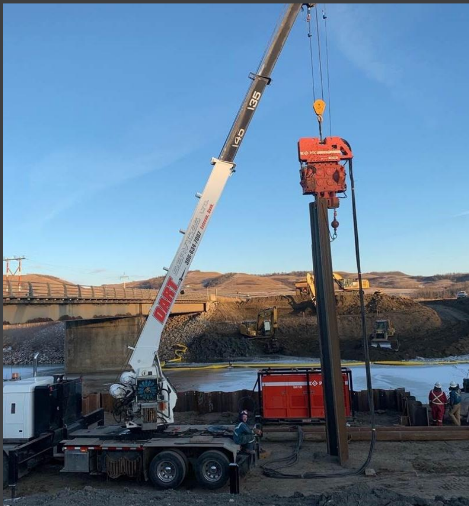
Driving 10 m AZ 26-700 double sheet piles.
