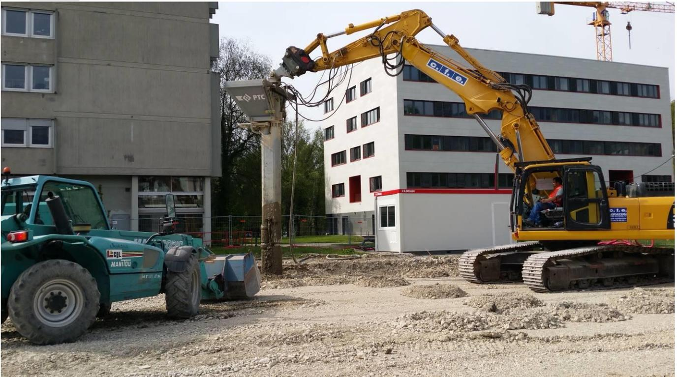
The gravel loader is a Manitou MT 1335, which is able to load the gravel into the tank and the bucket is adapted with a smaller opening in order to load the gravel on the front and all from the sides.
