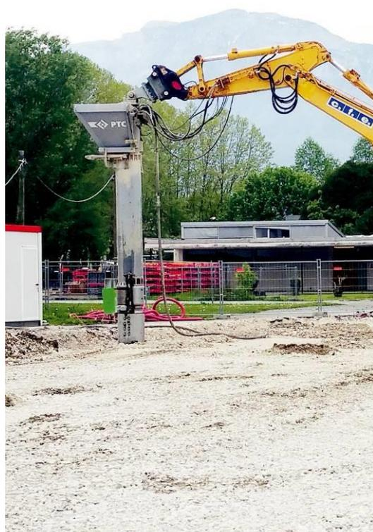
To improve the soil conditions, Franki Fondations used a Vibrolance VL18 with Bottom-feed system (BFS) for the installation and compaction of 850 stone columns of 4 to 6m deep.
